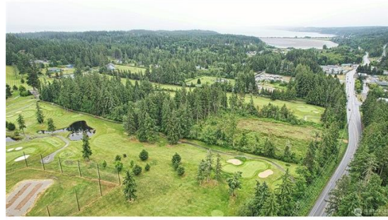
9.2 Acres Partially Cleared Looking South
